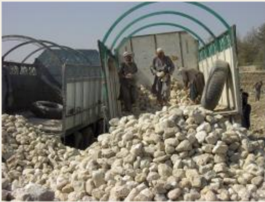
The first step in constructing a school.
